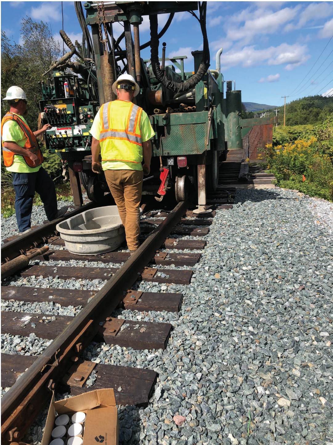
Figure B1: Boring B-4 Drilling (adjacent to the East Abutment)
