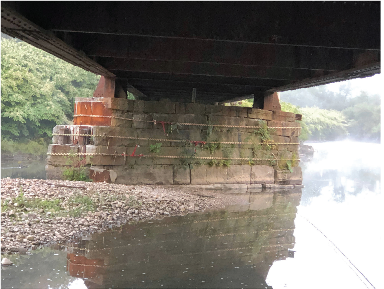
Figure B3: Existing Center Pier - Looking West from the East Abutment
