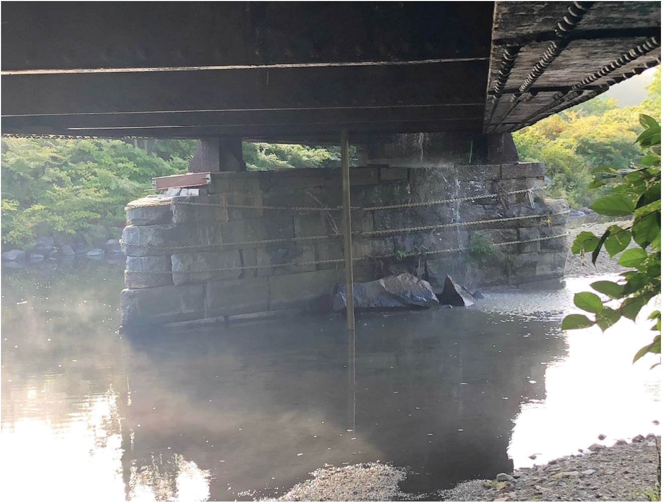
Figure B4: Existing Center Pier - Looking East from the West Abutment
