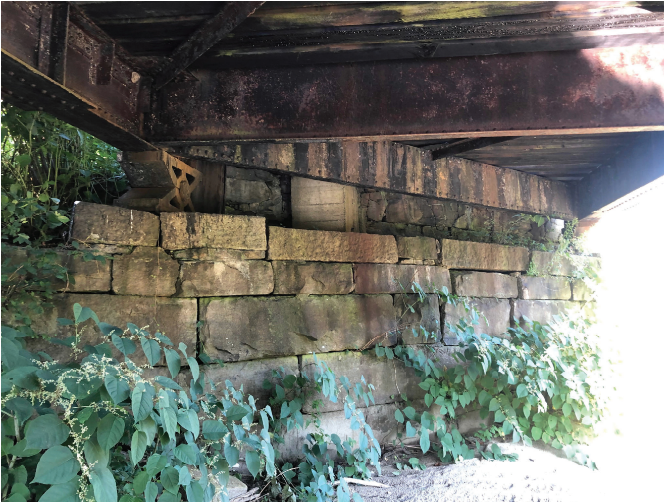
Figure B6: Existing West Abutment
