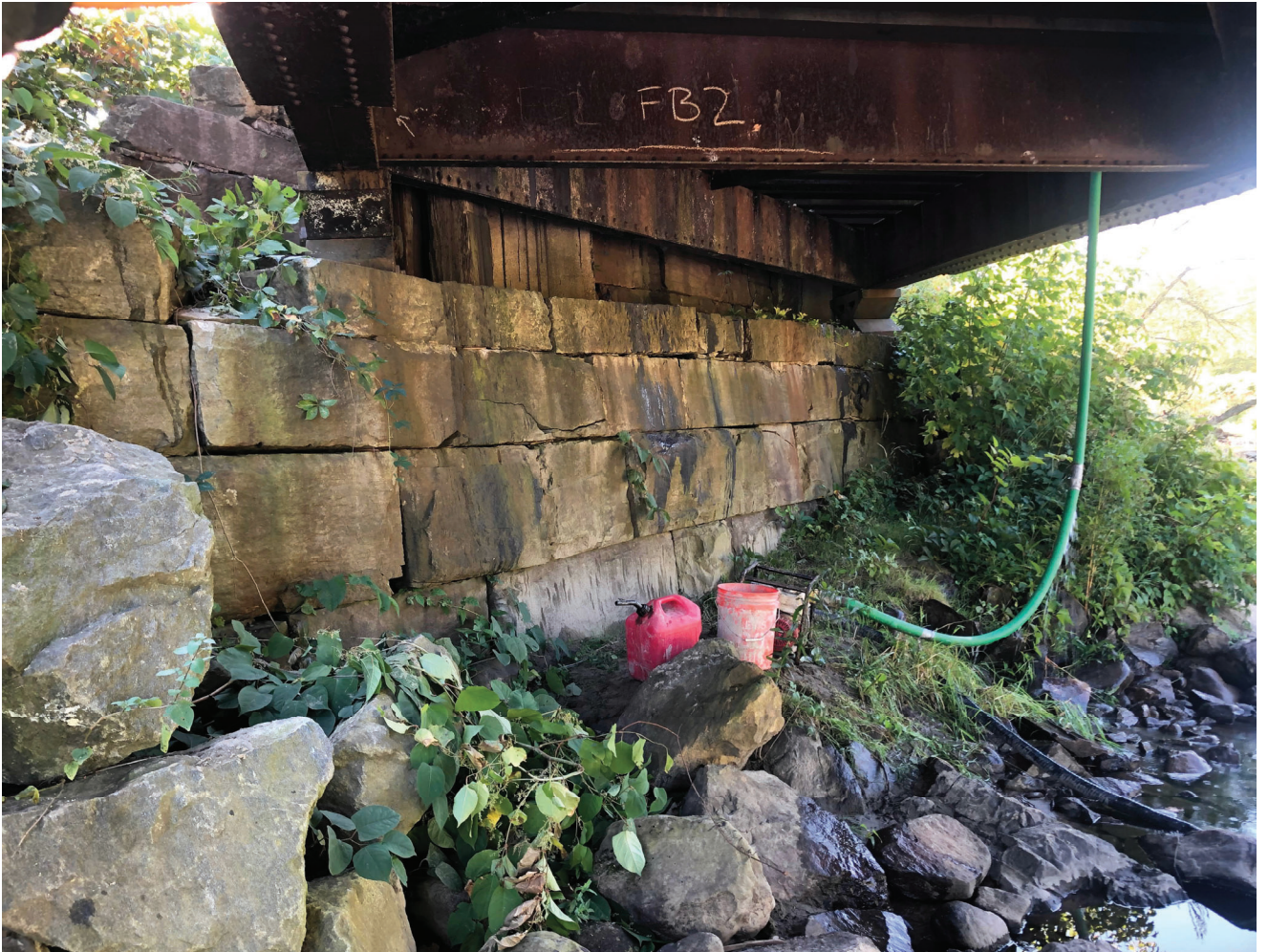
Figure B5: Existing East Abutment
