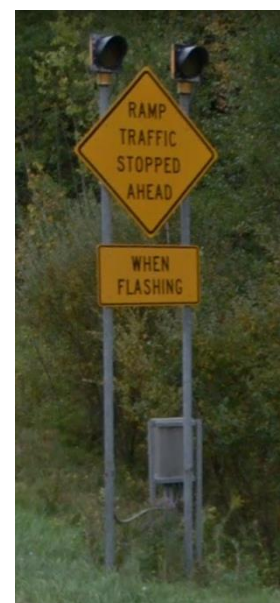
FIGURE 18: END OF QUEUE WARNING DEVICE IN ADVANCE OF EXIT 12 SB OFF-RAMP
