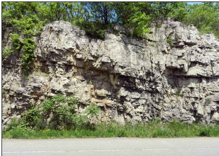
Figure 2: Photograph of westward facing rock cut along I-89 Interchange 16 northbound on-ramp. Note the presence of overhangs resulting from the deterioration along closely spaced jointing in the rock.
