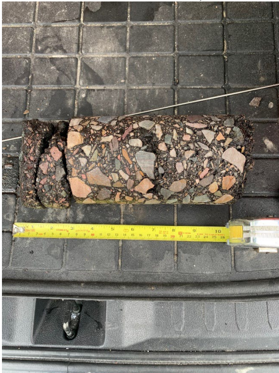
Asphalt core extracted at MM 61.0, Left Lane
