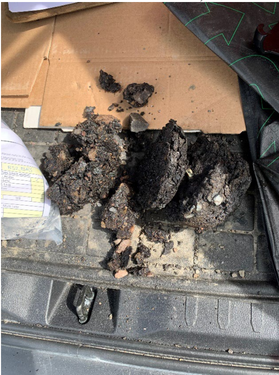
Asphalt core extracted at MM 60.0, Left Lane
