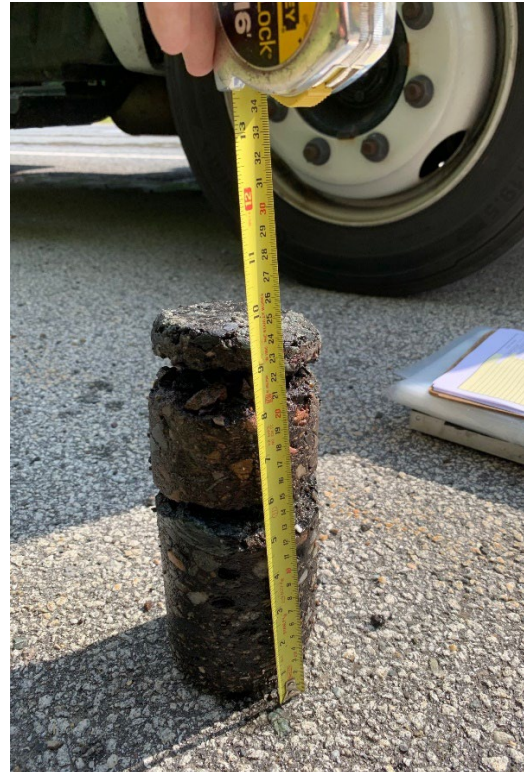
Asphalt core extracted at MM 63.0, Right Lane
