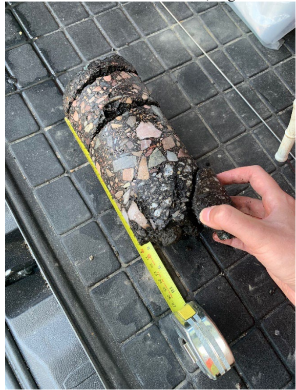
Asphalt core extracted at MM 61.0, Right Lane
