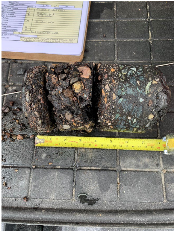
Asphalt core extracted at MM 59.05, Left Lane
