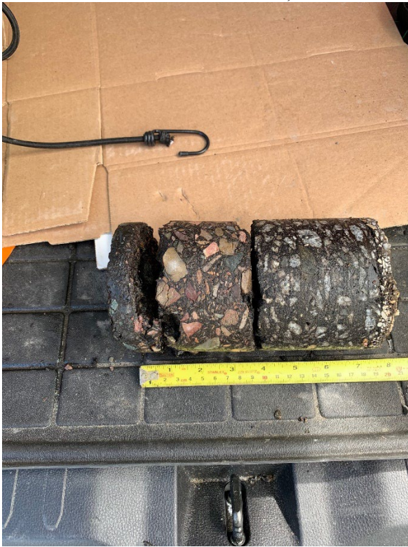
Asphalt core extracted at MM 56.0, Left Lane.
