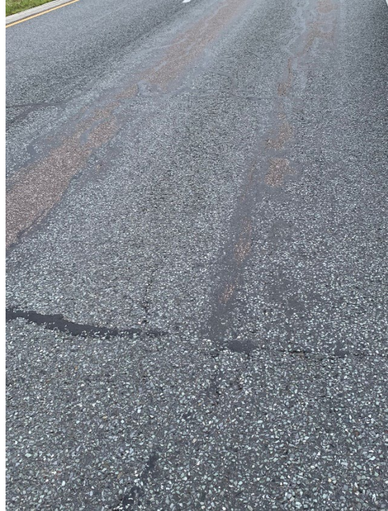
Surface Distresses at MM 56.0, Right Lane.
