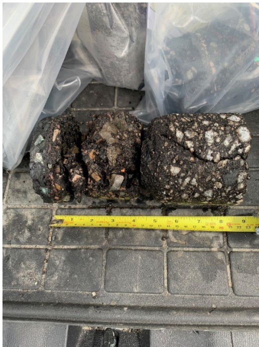
Asphalt core extracted at MM 54.0, Right Lane.
