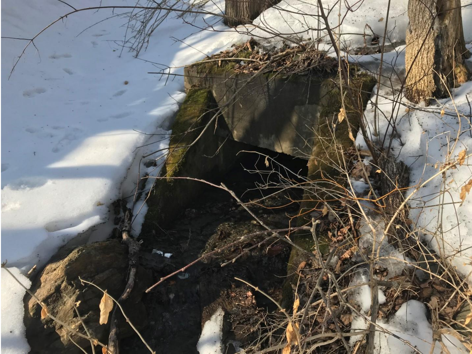
Figure 3: 3' x 3' Box Culvert at MM 6.0
